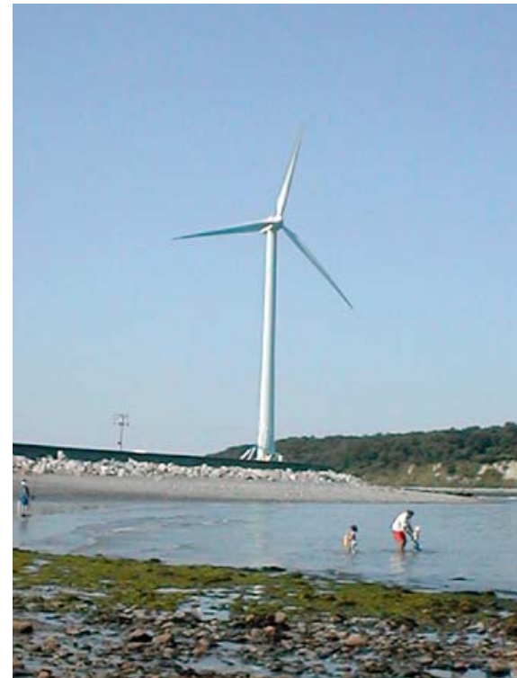
The 660 kW Vestas wind turbine in Hull, MA.
