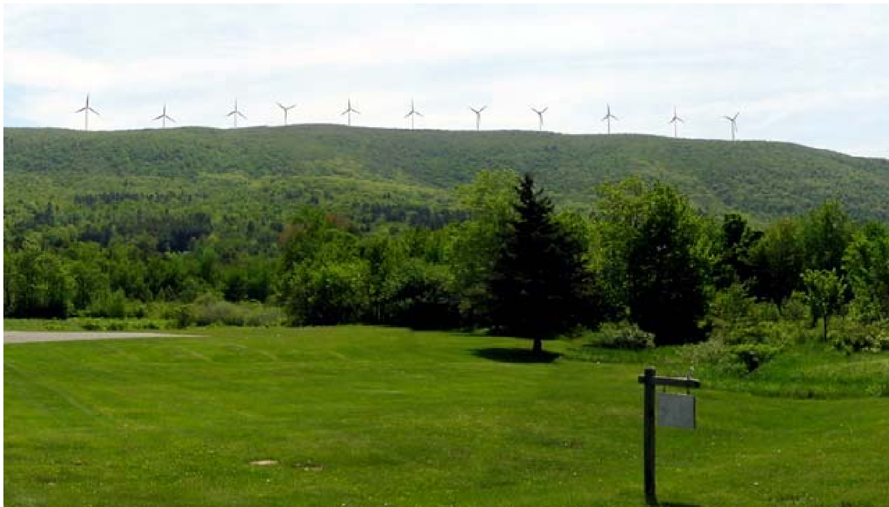
A visualization of the proposed Hoosac Wind project in Florida, MA. The project features twenty GE 1.5 MW turbines.
